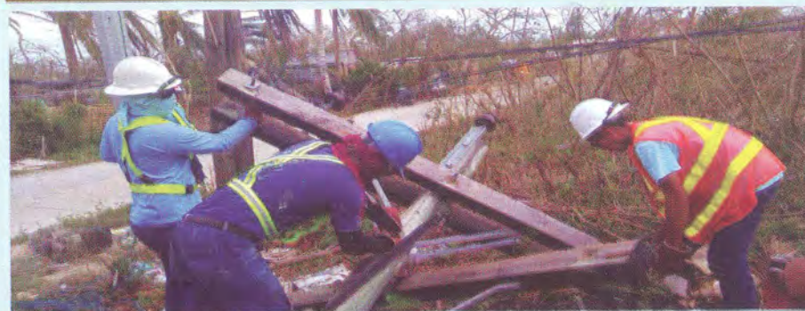
TOP: NEA sends off Task Force Kapatid (TFK) on December 1, 2016 for deployment in the areas hit by typhoon Lawin. BOTTOM: Volunteers of TFK-Nina repair a fallen pole within the coverage area of the First Catanduanes Electric Cooperative, Inc. (FICELCO).
